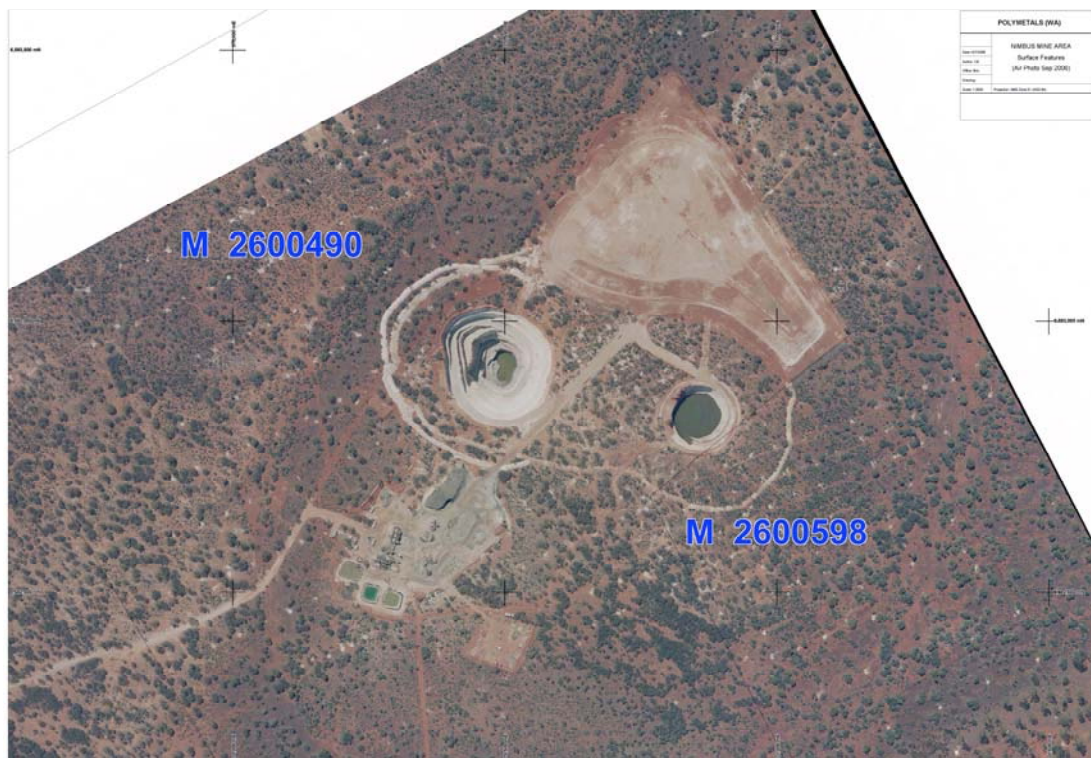
Figure 4. Processing plant, surface infrastructure and open pits at Nimbus project, within Mining Leases 26/490 and 26/598 (image courtesy: Polymetals Group Pty Ltd).
